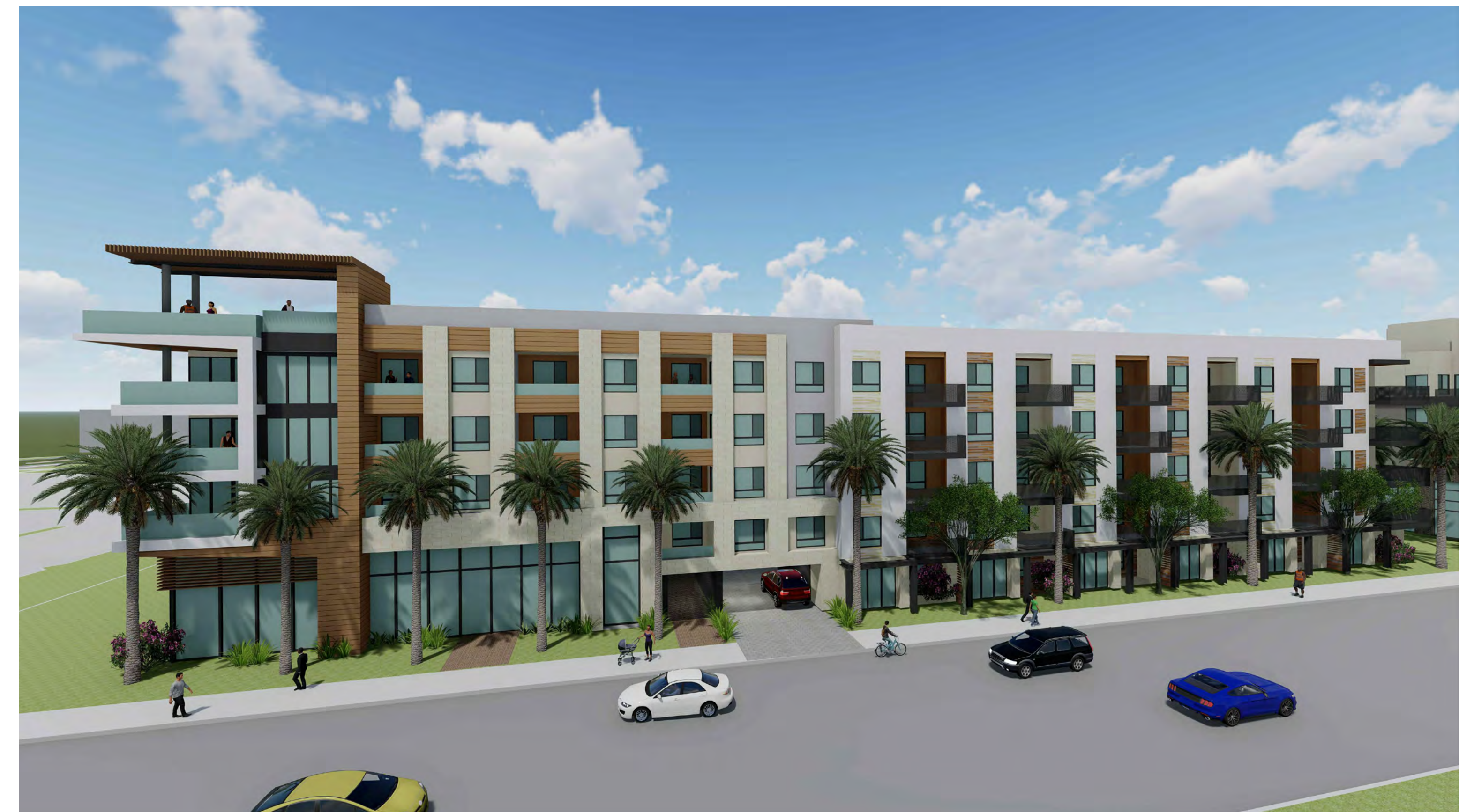
VIEW OF BUILDING B OPTION 2 (BUSINESS CENTER DRIVE)
